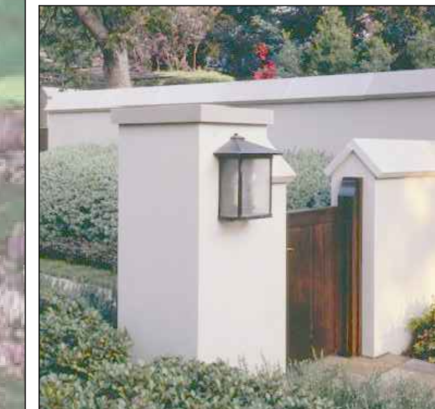
STUCCO WALL WITH STONE CAP
