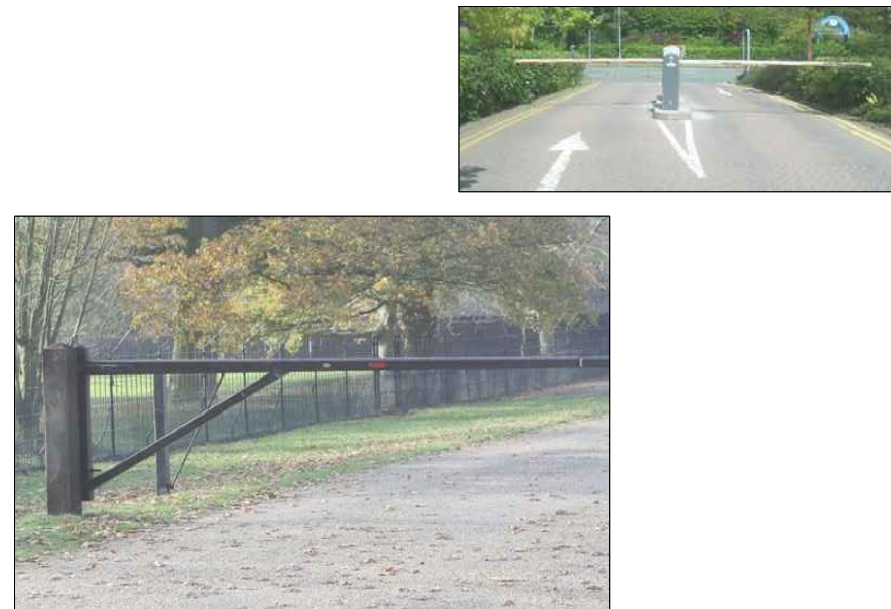
9 BARRIER ARM GATE
